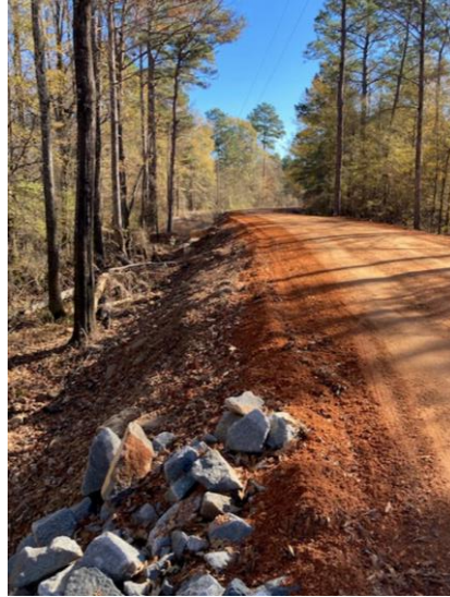
Figure 5: Elevated County Rd 303
