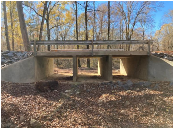
Figure 2: Triple 6x8x23 Box Culvert
