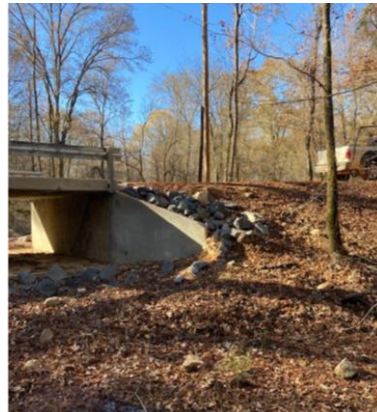
Figure 3: Rip Rap and Fabric on Slopes
