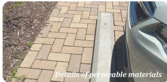
Permeable pavers in parking lot area
