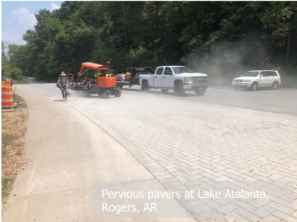
Pictured: 4G completing the mechanical installation of pervious pavers, Lake Atalanta, Rogers, AR.
