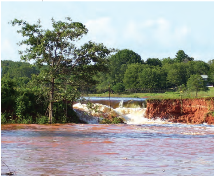
FIGURE 3.1 EMBANKMENT DAM FAILURE IN CLEVELAND COUNTY, OK
