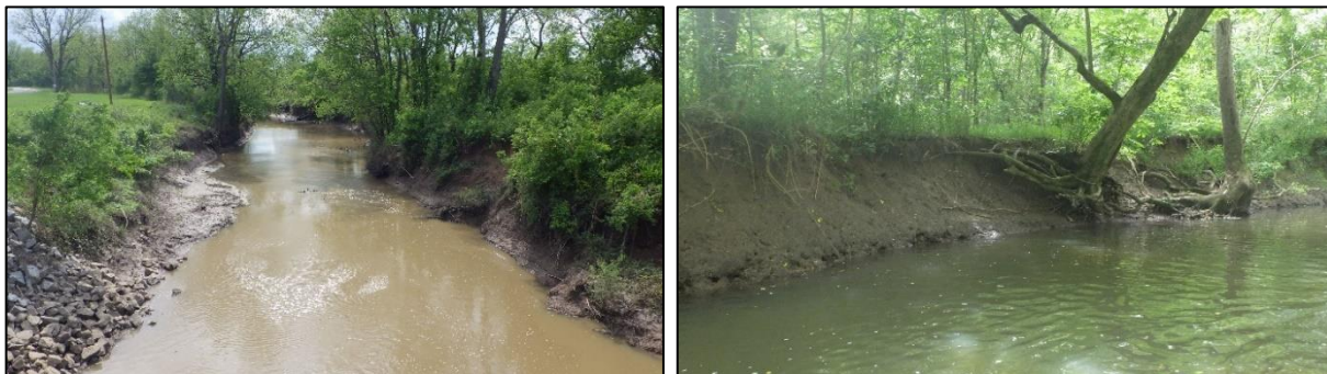
Figure 3.2.2. Streambanks with High Bank Erosion Hazard (left, SD-1;right, LC1).
