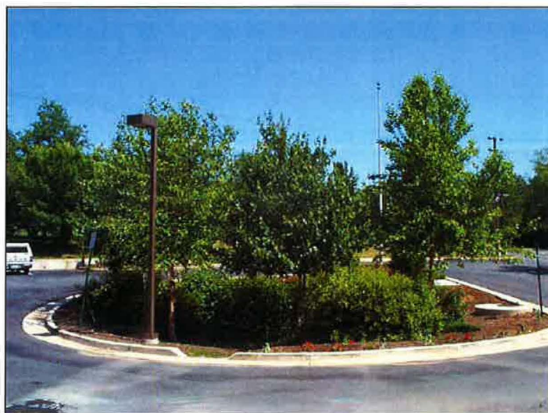
Figure 1: Bioretention created in a parking lot turn-around
